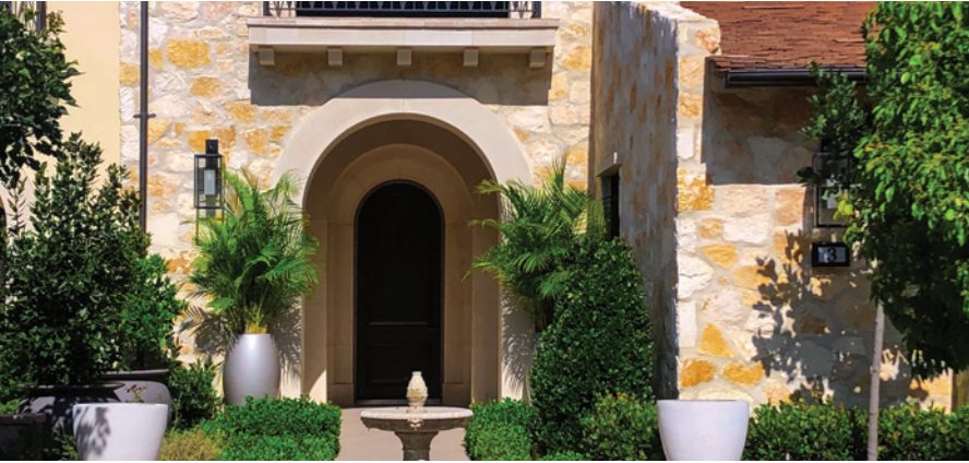
MONTGOMERY GOLD RUBBLE INSTALLED WITH A STANDARD RAKED MORTAR JOINT
