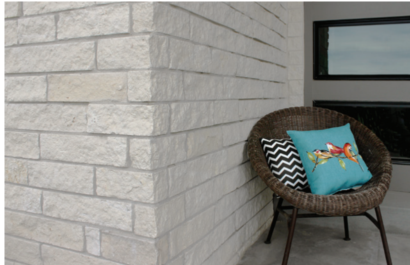
STELLA NEO LEDGE: SPLIT INSTALLED WITH A STANDARD RAKED MORTAR JOINT
