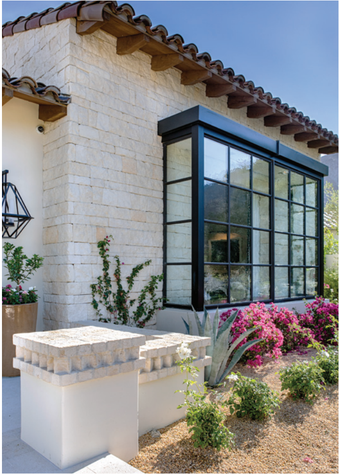
CAMILLA PILLOWED LEDGE INSTALLED DRYSTACKED
